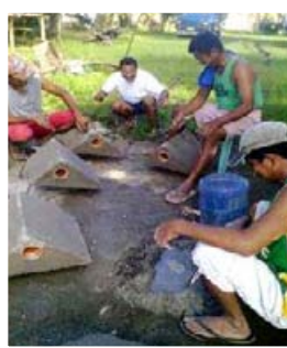
RC Metro Roxas: Production of the river crossing anchors for the Ameligan Matching Grant.
